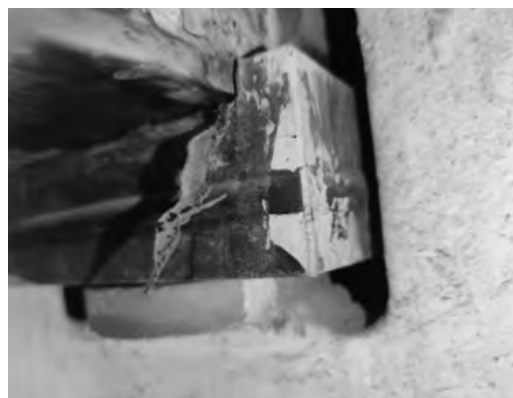
Figure 2. Expansion device sliding material grinding.
