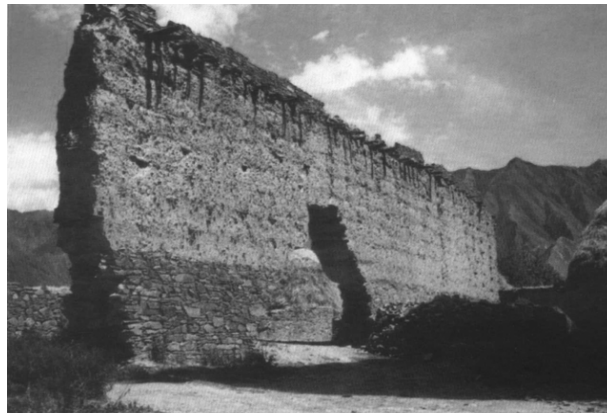
Figure 3. A protective wall of Nainingqude Temple (Image Source: Old house).
