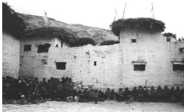
Figure 4. Benma grass stacked on the roof (Image Source: Old house).
